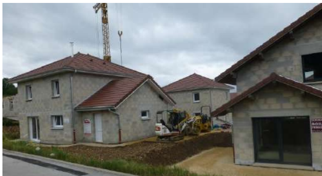
Construction neuve, Granges-Narboz
